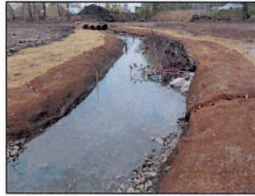
Figure 23. Log revetment / brush layering
