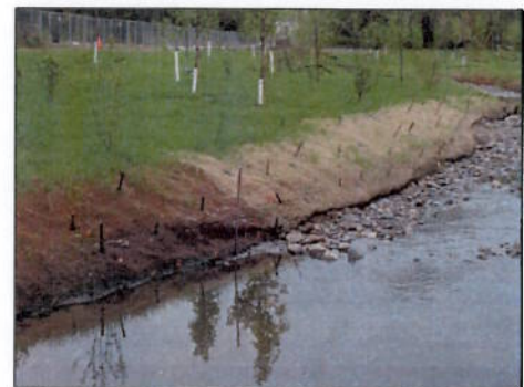
Figure 21. Live Stake Installed
