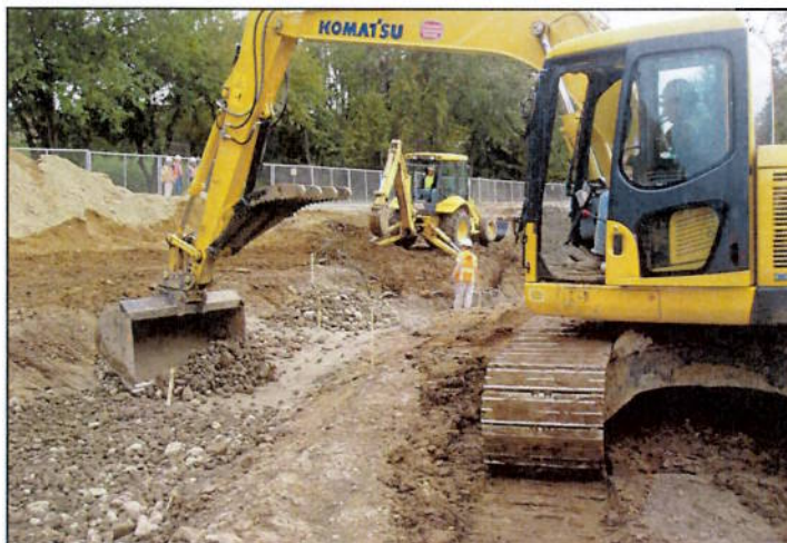
Figure 9. Substrate Installation
